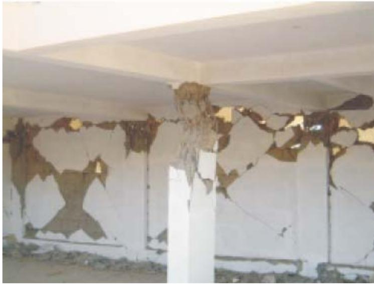
*Figure 2.7: Example of frame saved during the Bhuj earthquake by the presence of a few infills at the ground floor (Humar 2001)*
