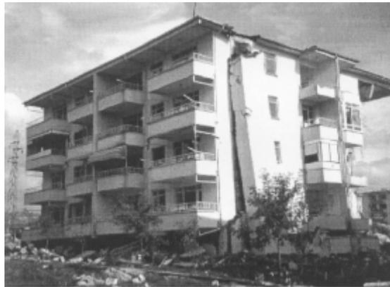
*Figure 2.5: Collapse of an uniformly infilled frame in its bottom two stories during 1999 Kocaeli earthquake (Dolsek 2000)*
