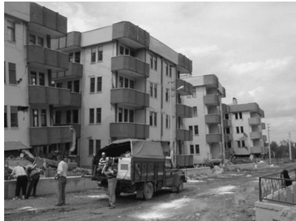
*Figure 2.6: Collapse of open ground story systems during earthquakes (Humar 2001, Scawthorn 2000)*
