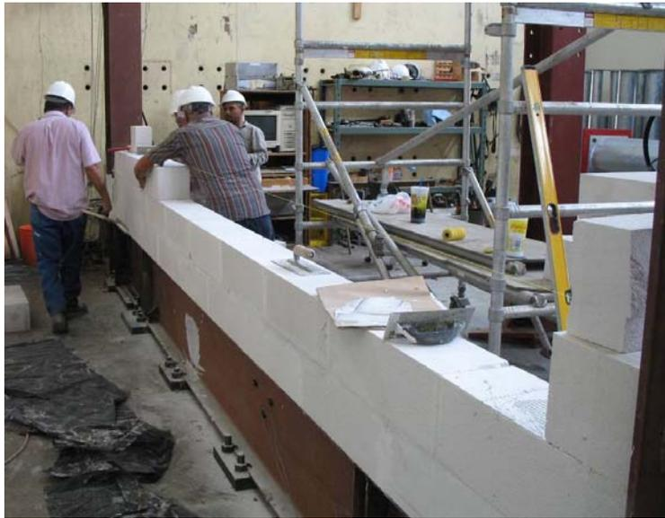
*Figure 4.10: Construction of AAC infill*
